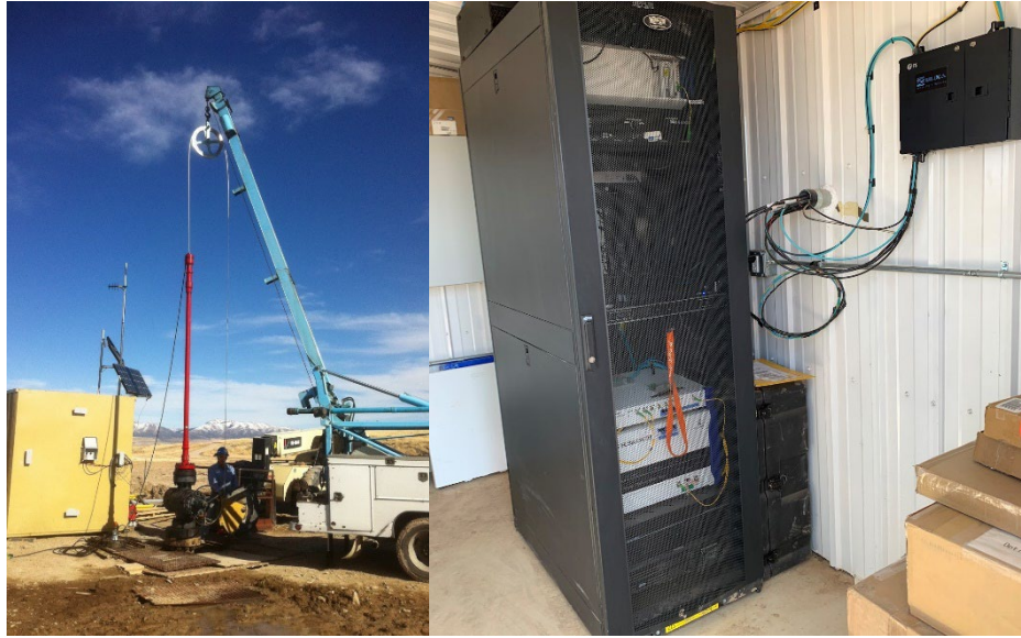
FIGURE E-8. DAS FIBER INSTALLATION AND INTEGRATOR
