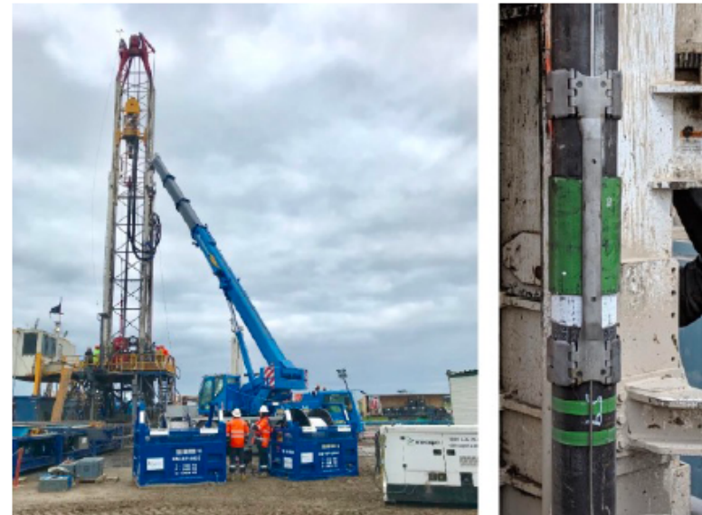
▲ FIGURE 12: A) Permanent cable installation on casing at CO 2 CRC site, Otway, Australia, and B) an example of a fiber optic cable installed along a steel casing with a cross-coupling cable protection.
