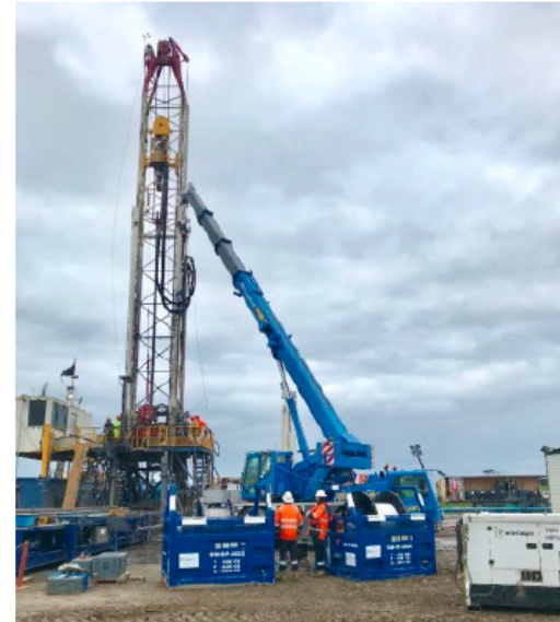
▲ FIGURE 12: A) Permanent cable installation on casing at CO2CRC site, Otway, Australia, and B) an example of a fiber optic cable installed along a steel casing with a cross-coupling cable protection.
