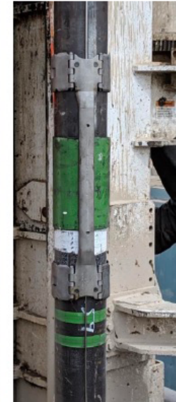
▲ FIGURE 12: A) Permanent cable installation on casing at CO2CRC site, Otway, Australia, and B) an example of a fiber optic cable installed along a steel casing with a cross-coupling cable protection.
