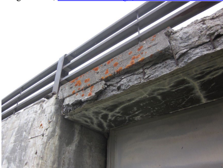
Figure A.II-1.3-1. Highway Bridge with Spalling Concrete and Rusting Rebar
