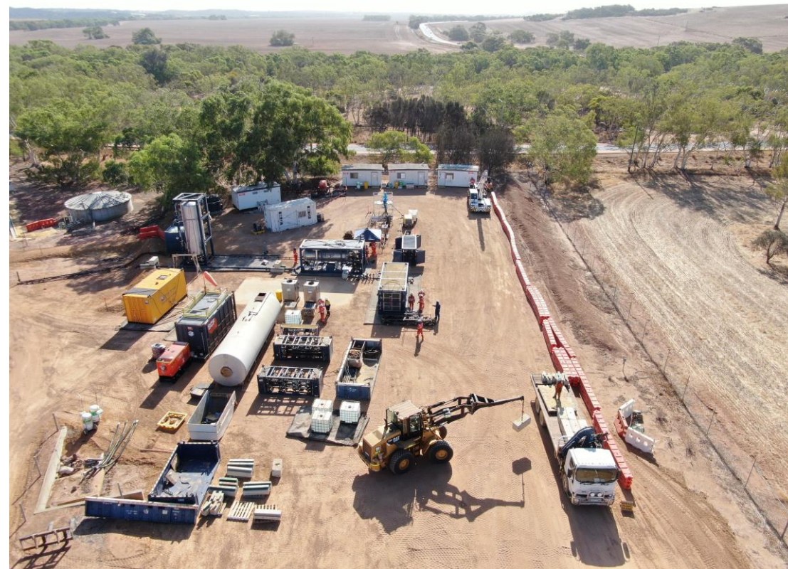
Inject truck-supplied CO2 in the Dongara reservoir
