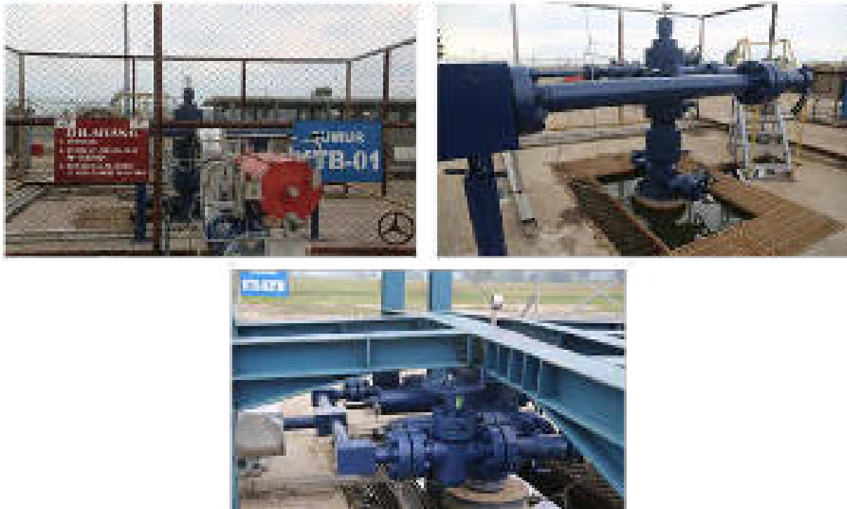
Figure 20: KTB-01 & KTB-03TW Wellheads
