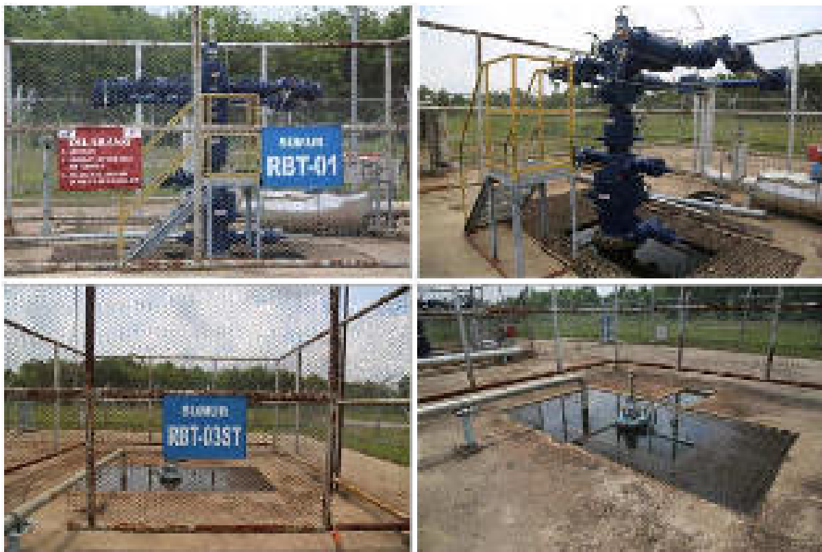
Figure 6: RBT-01 and RBT-03ST (water injection) Wellheads
