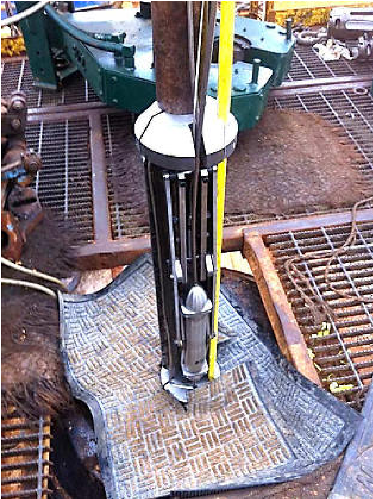
Figure 11 Typical Geophone and Flat Pack Installation on CO 2 injection tubing.
