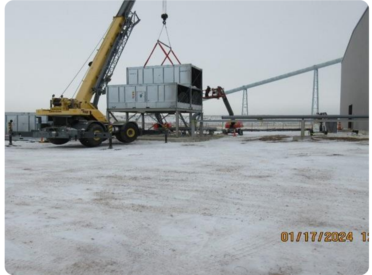
Evaporative Cooling Tower
