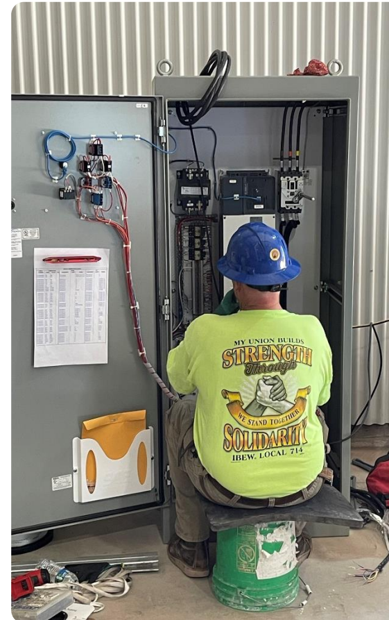
Electricians terminating cables
