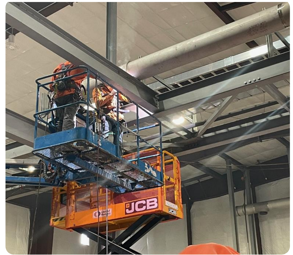
Installing process piping
