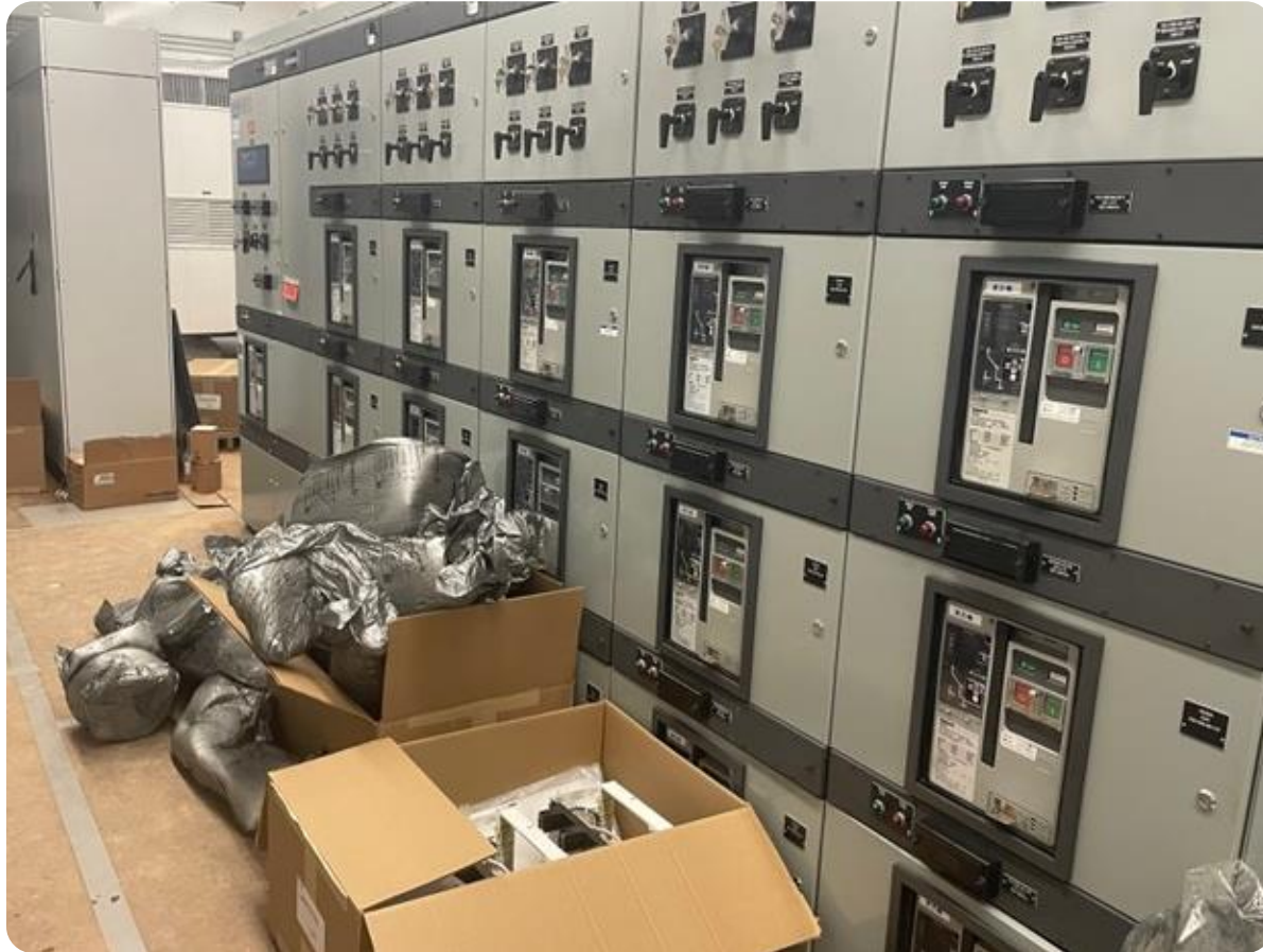
PDC Interior – electrical switchgear and motor controllers
