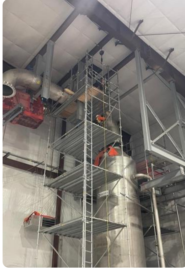
Direct Contact Cooler - April
