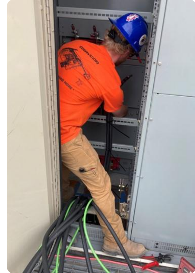
Electricians terminating cables
