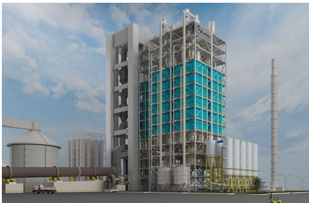
Figure 3: An impression of a Leilac plant at typical full-scale. Capable of capturing ~600 000 tonnes of CO 2 per year, with a footprint of 54 x 27m and height of 90m.
