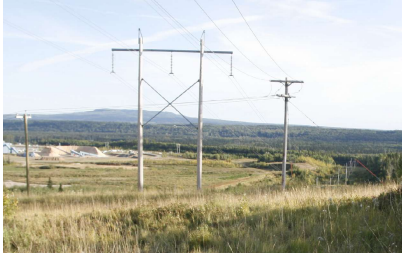
Existing H-frame 240 kV transmission line in the area (foreground of photo)
