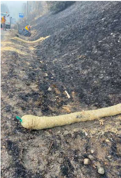
Photo 1. Erosion sock for sediment erosion control
