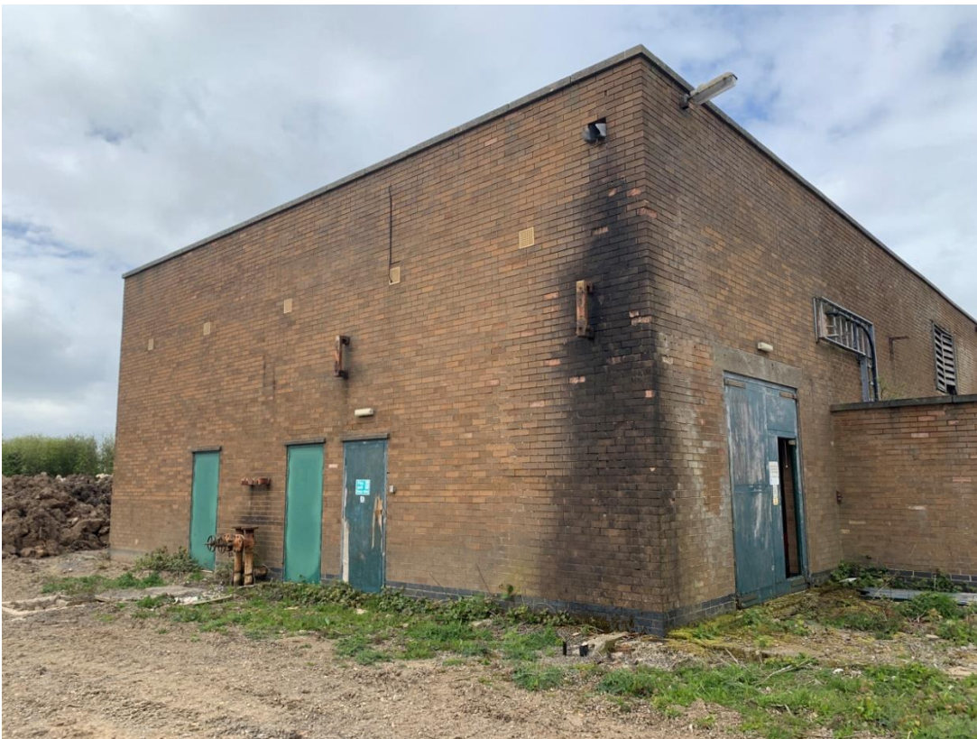
Photograph 2. Derelict building identified within the Main Site.
